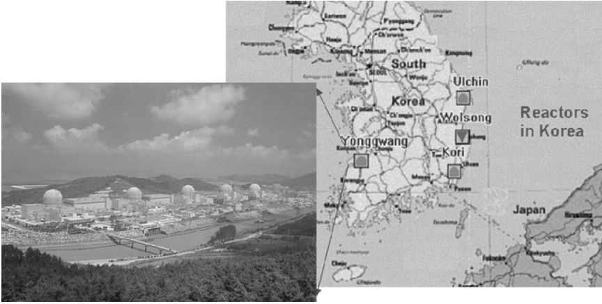
Fig. 1 Overview of Yonggwang nuclear power plant and location of the plant.
